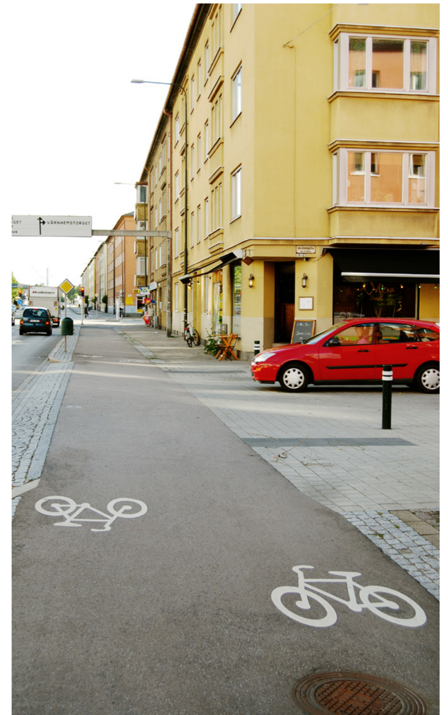
Connecting local street with speed limited cycle lane running along the entire street, Nobelvägen, Malmö.
