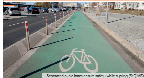
Separated cycle lanes ensure safety while cycling (© QIMBY)
