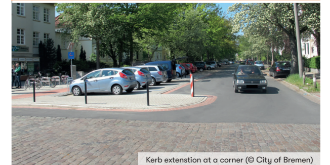
Kerb extension at a corner (© City of Bremen)
