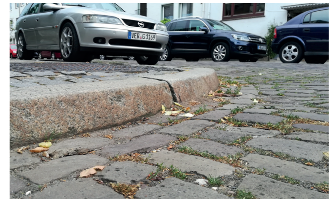
High curbs and cobblestones in the streets of the Hulsberg neighbourhood. Source: S. Findeisen, City of Bremen
